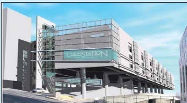
RTKL Associates is converting its offices to Autodesk Revit after experiencing the benefits of building information modeling on major projects such as this Washington DC Union Station Garage addition.
